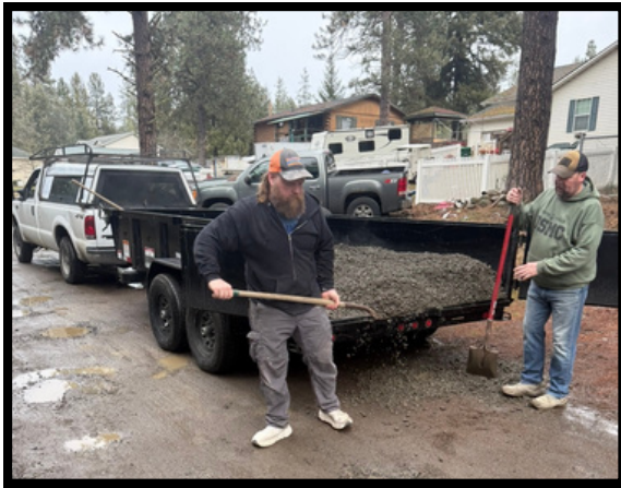
Keith Cox and Ben Bersegal filling potholes
