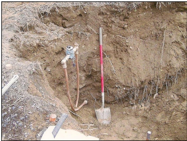
Newly installed meter, ready for back fill.
