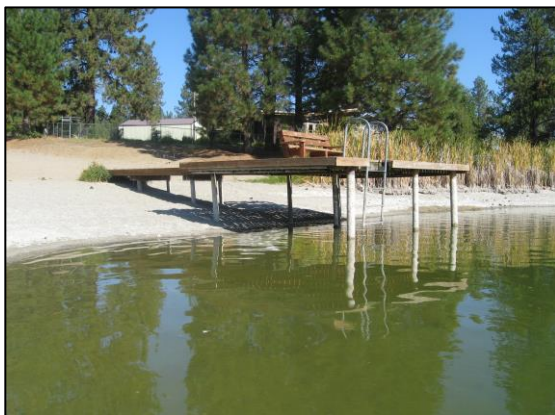
Bing's Landing dock with exposed steel pilings, 2011.
