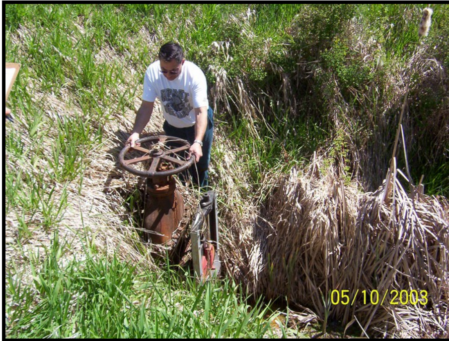
Carl Hockhalter opening and testing the south dam foot valve.
