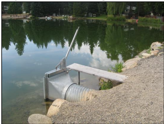
John Fechner designed new fish screens.
