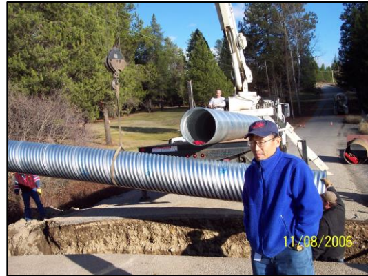
Dam Safety Officer inspecting work.
