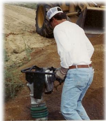
Carl working the compactor
