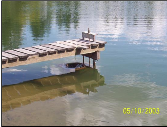
Defective trickle tube was removed.
