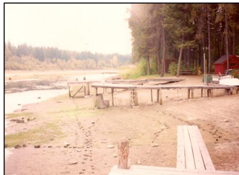
After 40 years Russell is replaced the dock in 2011. The end of the original dock was built on a large stump.
