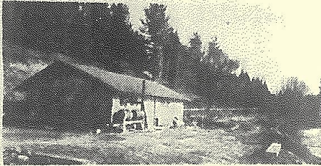
Newly constructed modern hatchery at Reflection Lake showing water pipe from spring. More than 1,000,000 trout will be reared here this year.
