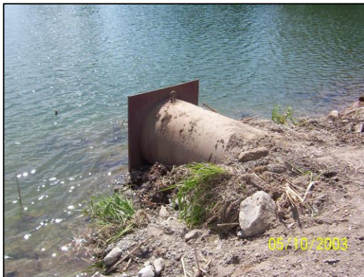
Original 36" overflow replaced.
