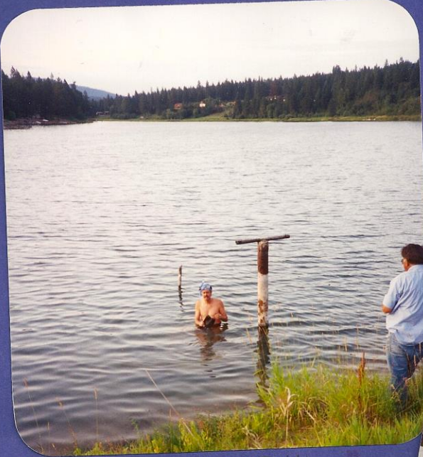
MARK Wiser & Pat Rickey Checking South Dike inside valve.
