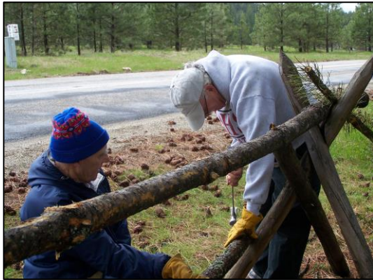
Lee Osborne and Jerry Parker building a rail fence above the center.
