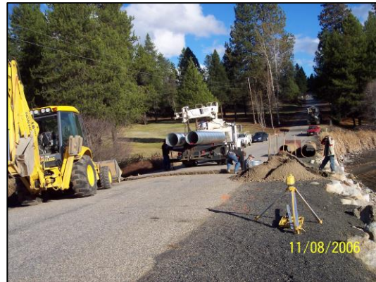
Replacing 36" overflow in 2006.
