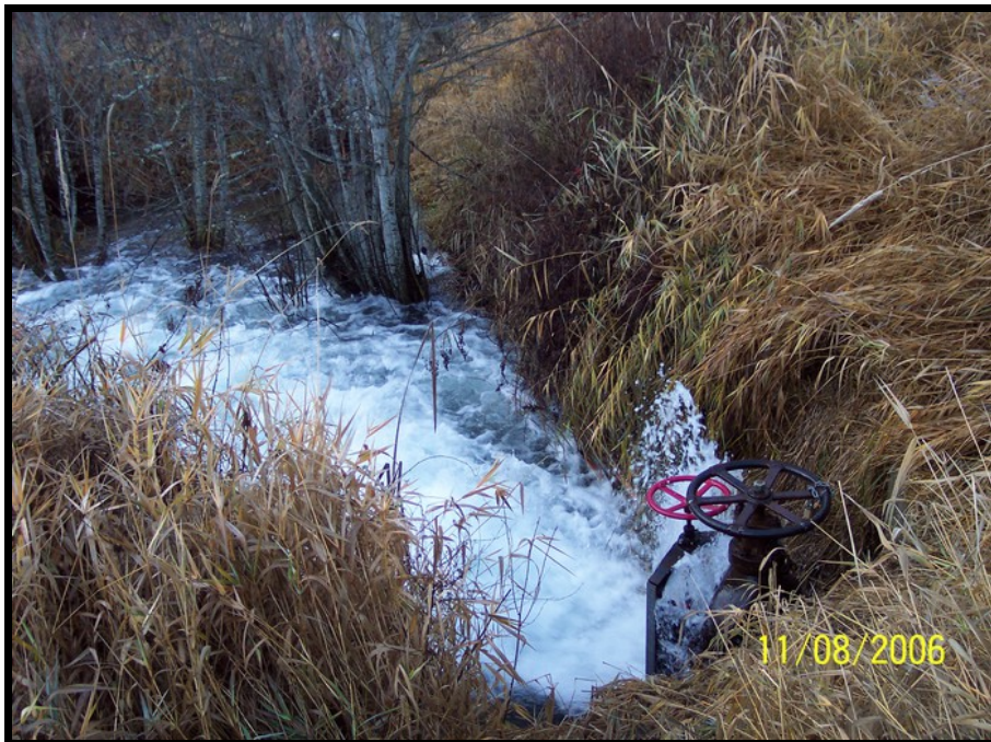
Foot valve is often opened in the fall to lower the lake for maintenance.
