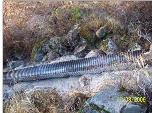
Concrete re-enforces overflow.
