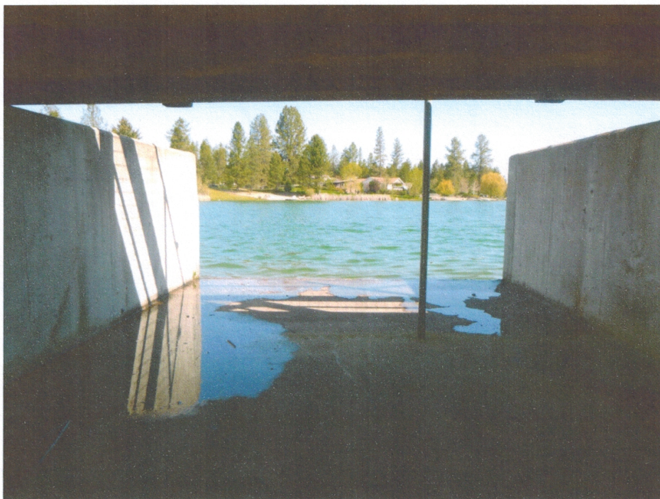
Photo 10: Emergency Spillway Entrance on South Dam
