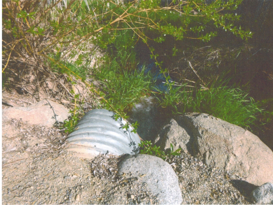
Photo 13: Auxiliary Spillway Discharge on North Dam
