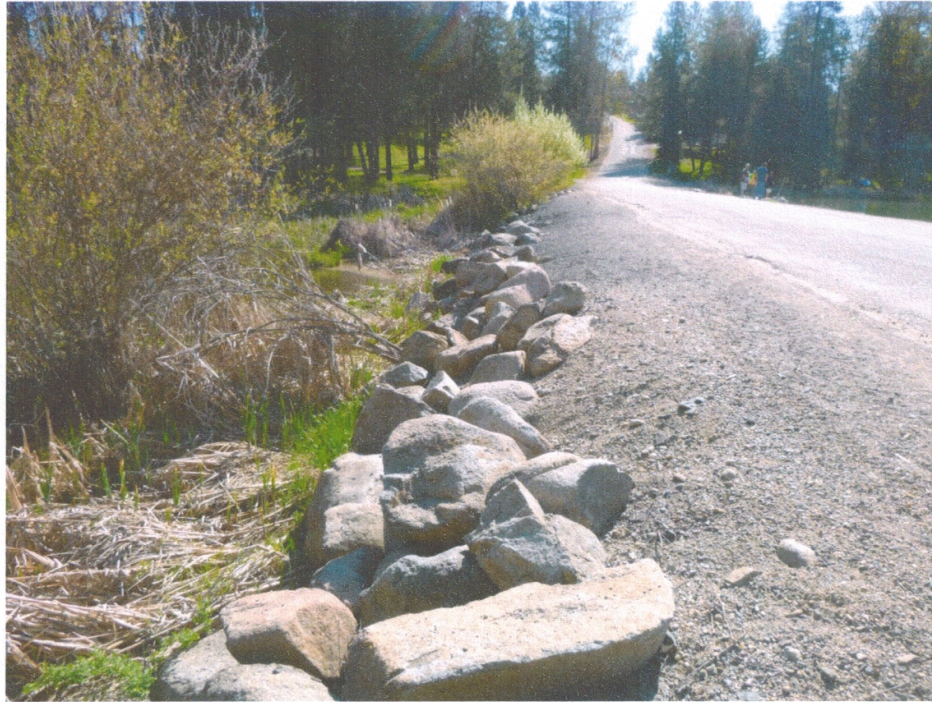
Photo 7: Reflection Lake North Dam - downstream face
