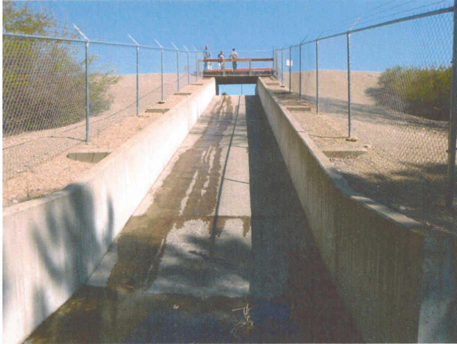
Photo 11: Emergency Spillway on South Dam, looking upstream
