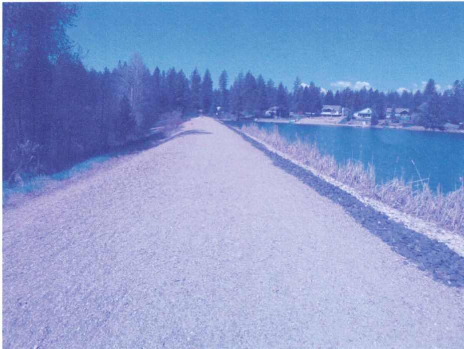
Photo 2: Reflection Lake South Dam - crest
