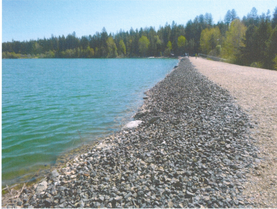
Photo 3: Reflection Lake South Dam - upstream face
