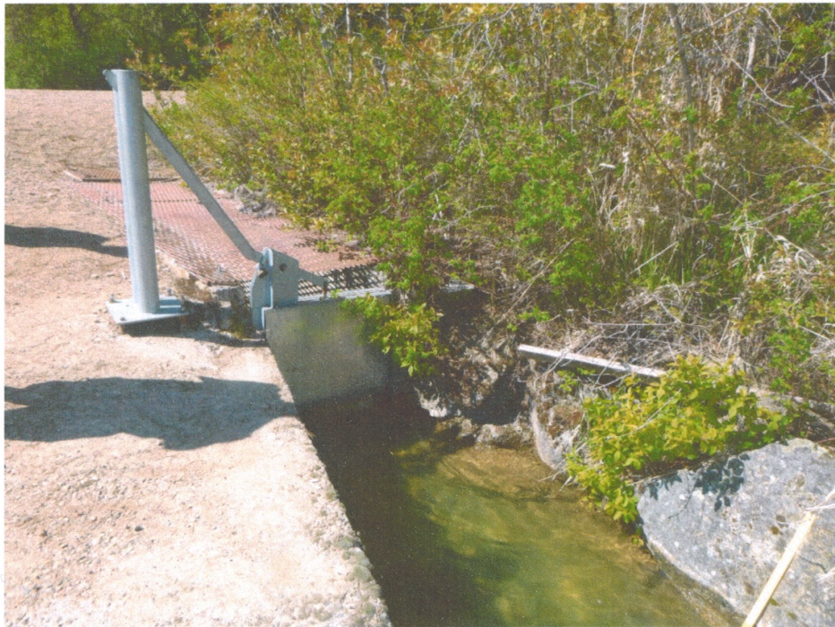
Photo 8: Principal Spillway Entrance on South Dam
