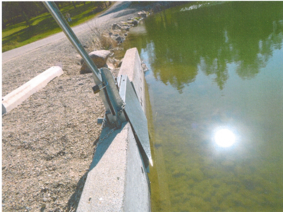
Photo 12: Auxiliary Spillway Entrance on North Dam
