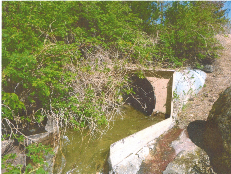
Photo 9: Principal Spillway Discharge on South Dam
