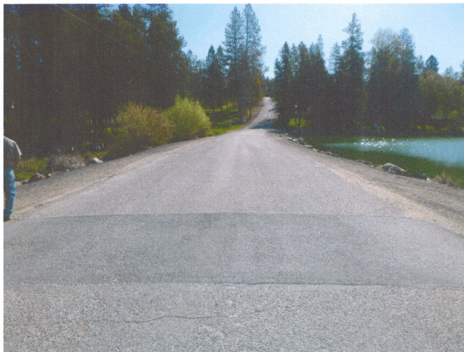
Photo 5: Reflection Lake North Dam - crest
