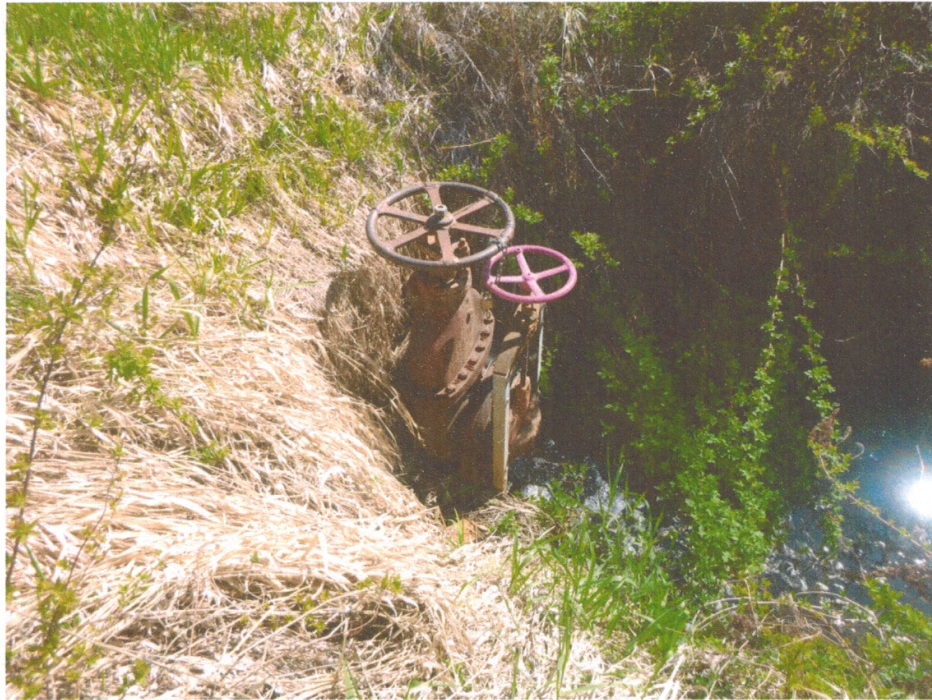
Photo 14: Low Level Outlet on South Dam
